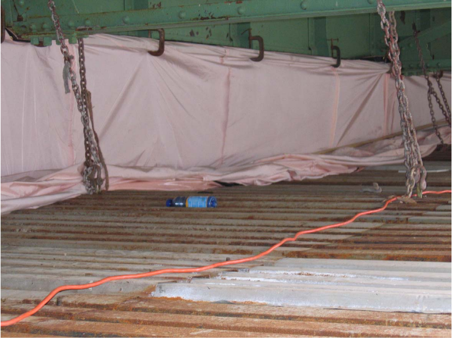
Cable Supported/Metal Deck Platform System & Side Containment
