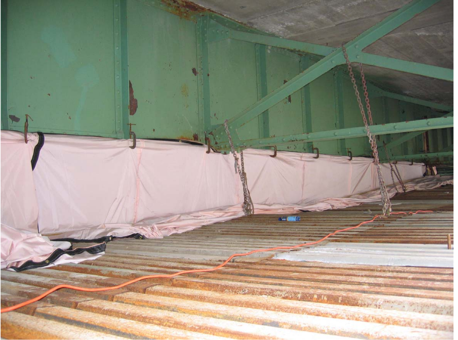
Cable Supported/Metal Deck Platform System & Side Containment
