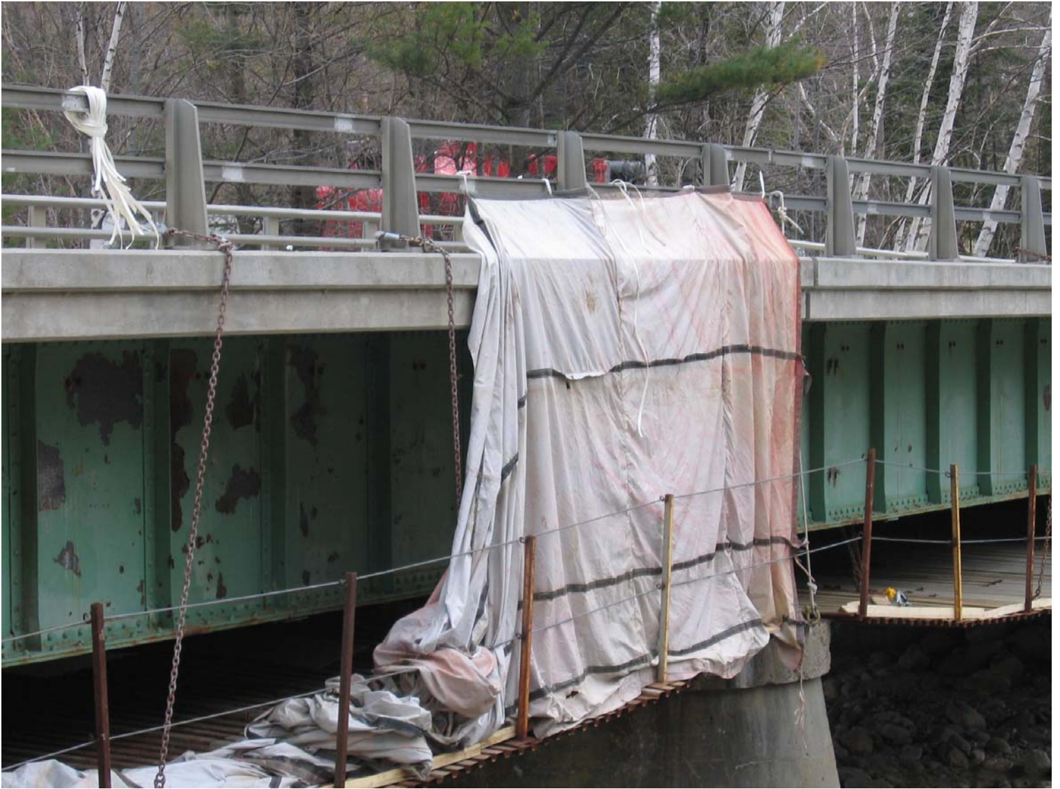
Cable Supported/Metal Deck Platform System & Containment
