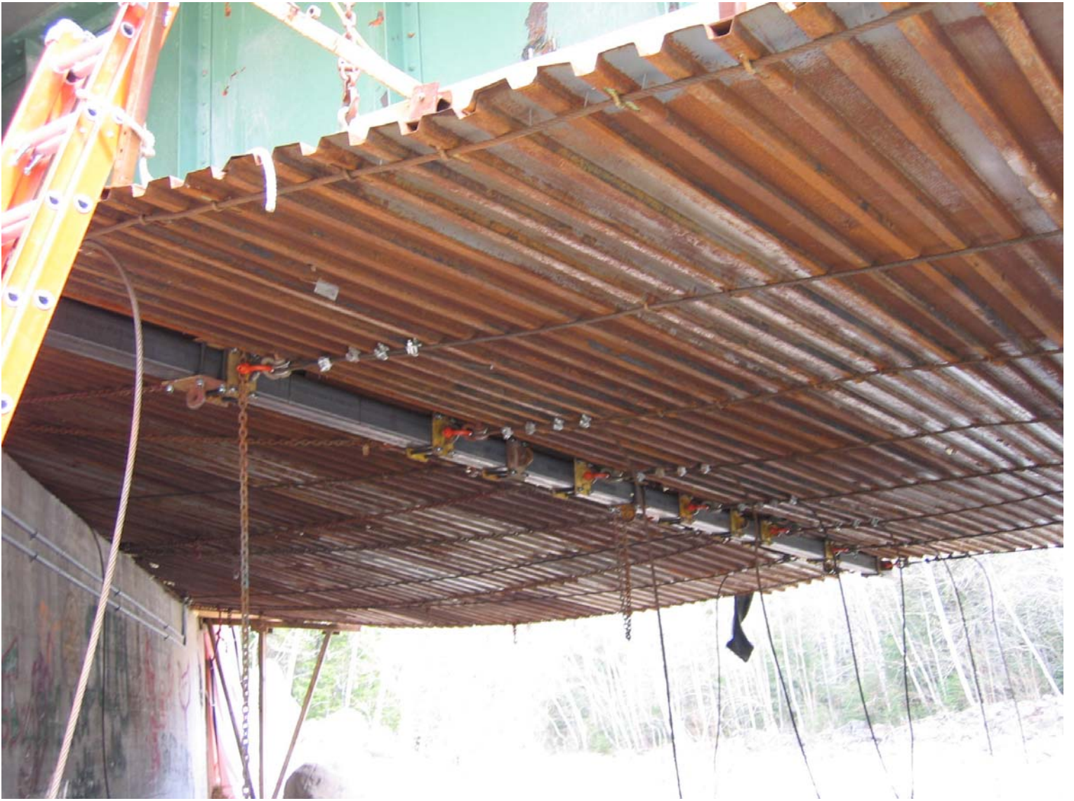
Horizontal End Support Beam Assembly W/ Clamping Plate Assemblies & Chain Tie Backs & Cable Supported/Metal Deck Platform System
