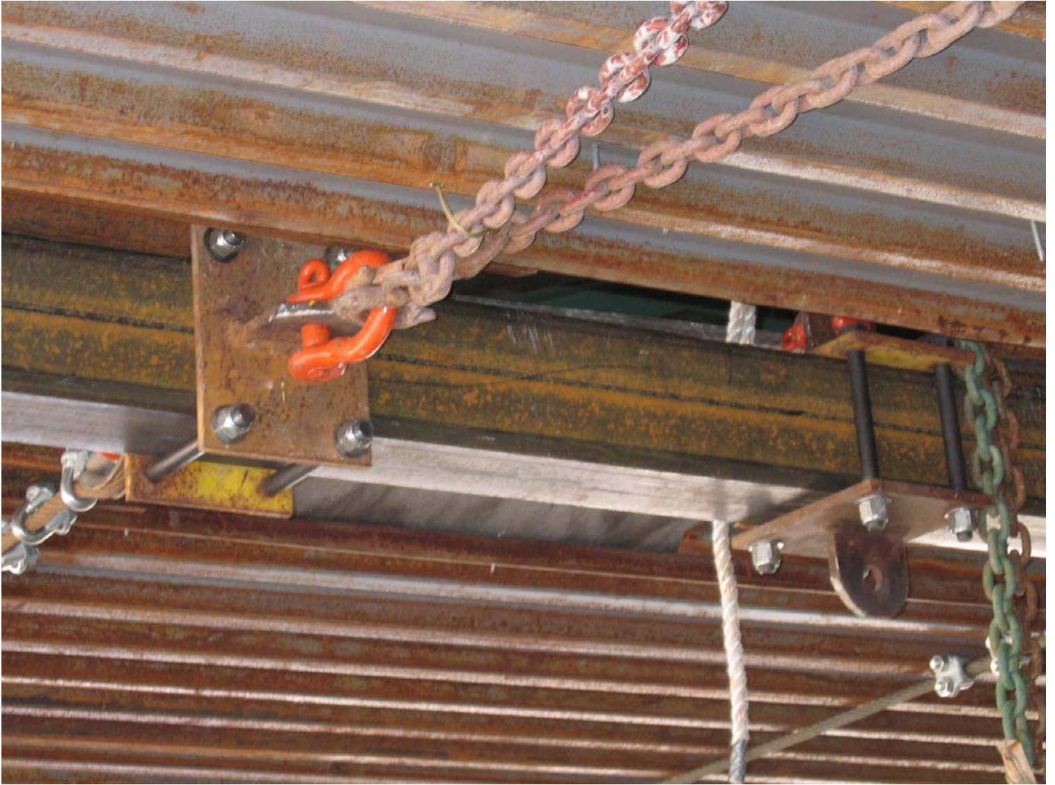
Horizontal End Support Beam Assembly W/Clamping Plate Assemblies & Chain Tie Backs
